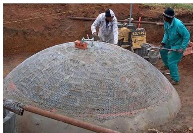
Figure 18. Fixed Dome Digester During Construction
