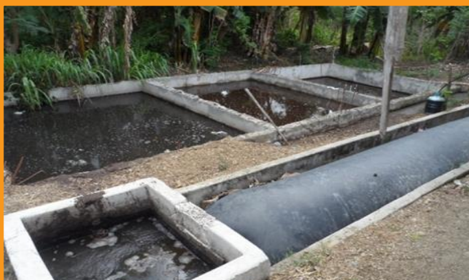
Mixing Pit (top) and Tube Digester (bottom)
