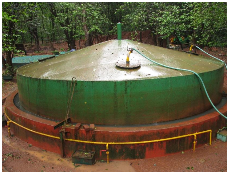
Figure 22. Floating Drum Digester
