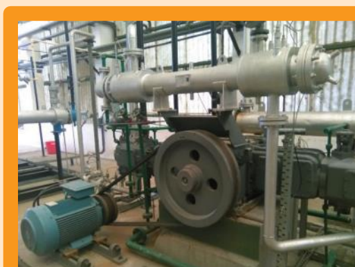
Biogas engine genset
